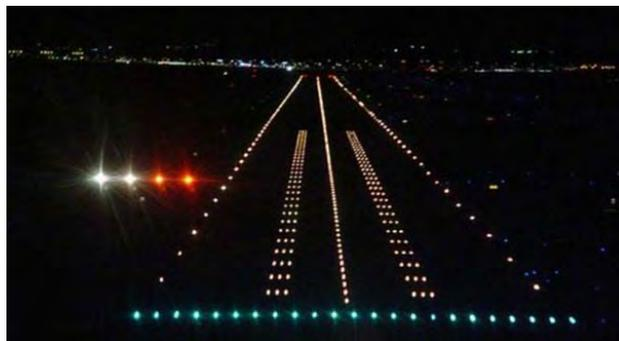
Figure 4.1 - PAPI lights to the left of the runway lights. Two red and two white lights as pictured indicate the nominal approach path. Notice the red lights are of lower intensity
